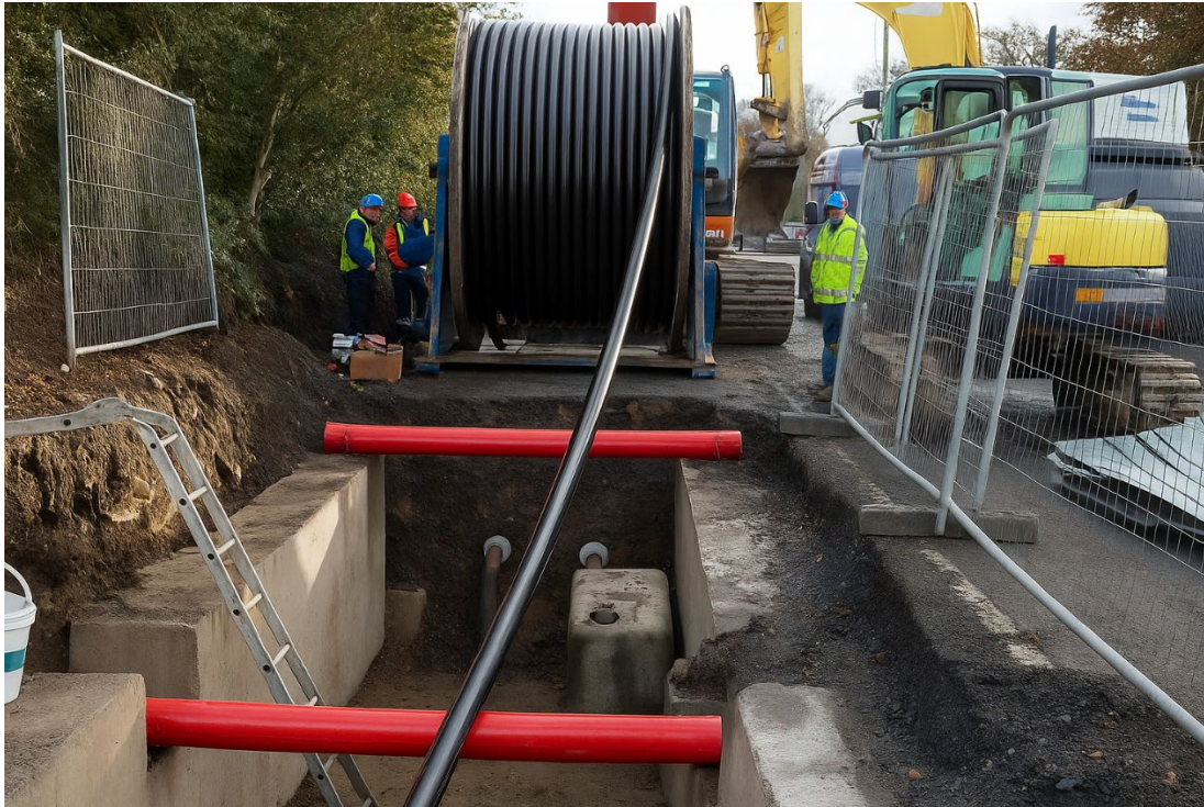
Figure 13: HV cable pulling procedure (Typical drum set-up)
