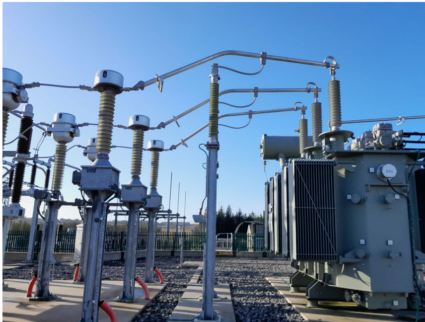
Figure 8: Typical 110kV Transformer Connection
