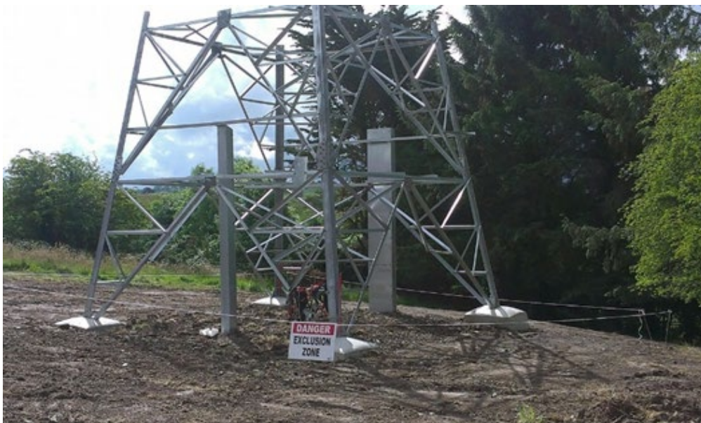
Figure 4: Base of End masts Structure Backfilled
