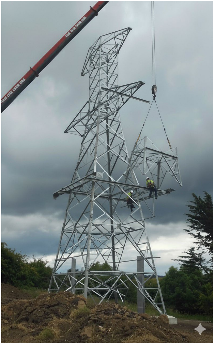
Figure 5: Cable End Mast
