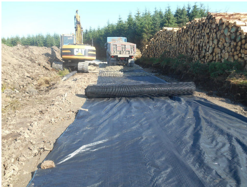
Figure 15: Access Track Build-up with Geotextile
