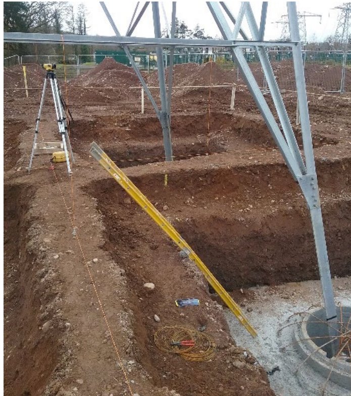
Figure 3: Typical 110kV end masts foundation excavation
