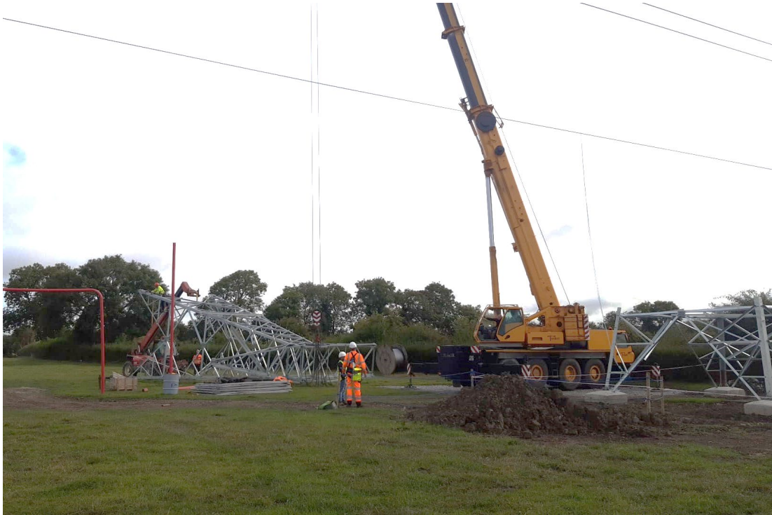
Figure 16: Crane pad and laydown areas
