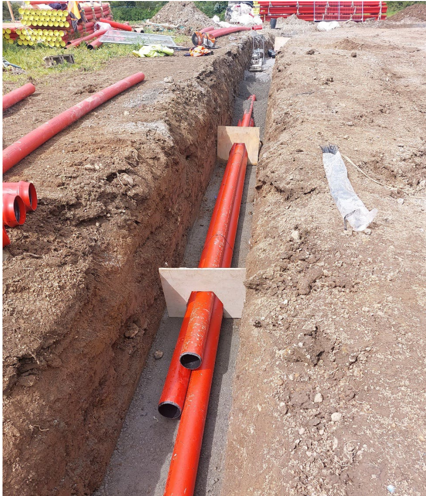
Figure 9: Typical 110kV Underground Duct Installation on Private Land
